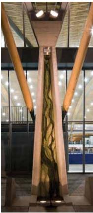
To light the art in the concrete buttresses. two in-ground uplights were recessed in the gutter. Two concealed CMH spotlights mounted on both sides of the downspout also graze the carvings
